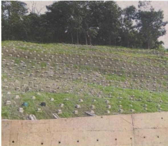
DBKL has installed beam grids on slopes in Jalan Kasah to strengthen them.
